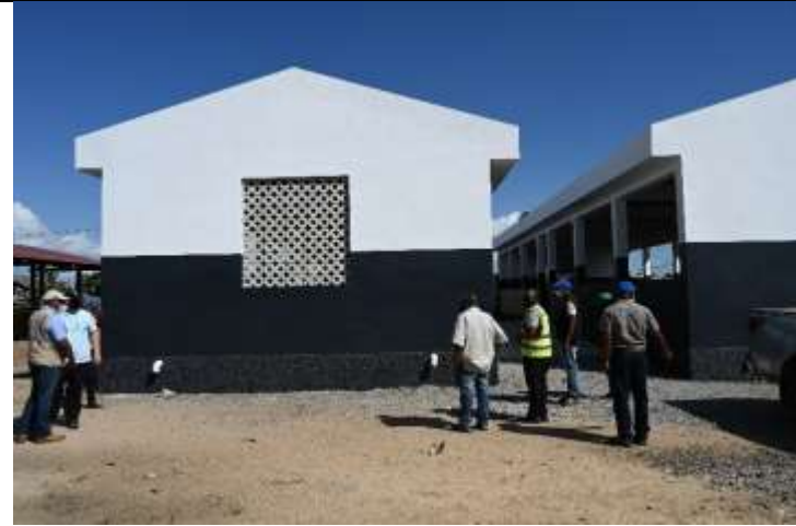
Picture 2 shows newly constructed two market blocks in Tica, Nhamatanda
