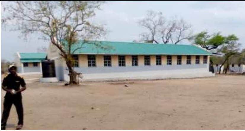
Picture 7 shows that the newly constructed school block-1 with gender friendly toilet behind the school in Chicuacha, lot1, Chibabava district.
