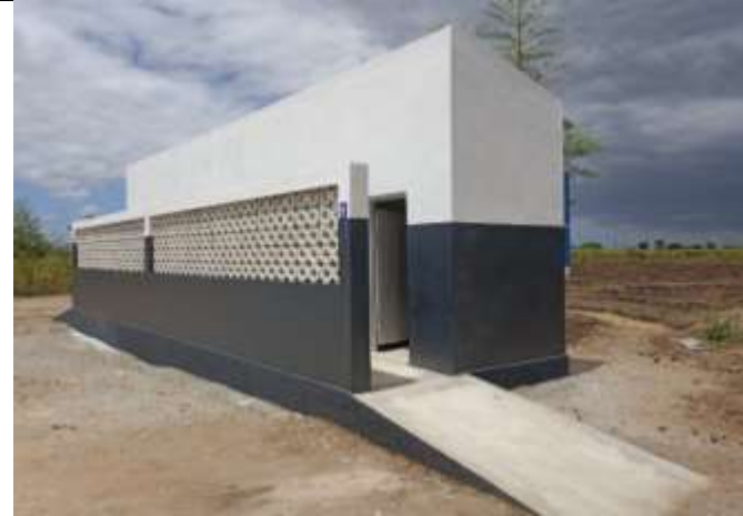
Picture 12 shows newly constructed gender friendly toilet (front view) in Guara Guara Buzi
