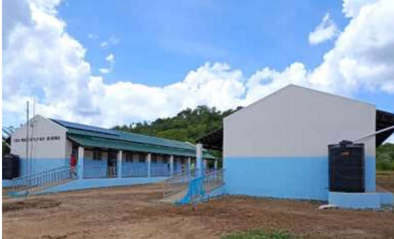
Picture 15 shows newly constructed schools in Muconja, lot2, Chibabava district.
