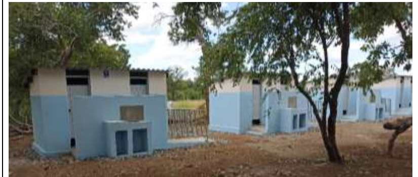
Picture 20 shows newly constructed gender and disabled friendly toilets in Armando Emilio Guebuza, lot3, Chibabava district.
