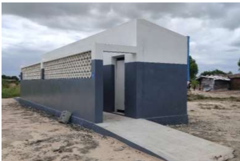
Picture 7 shows newly constructed isometric view of gender friendly toilet in Mutua
