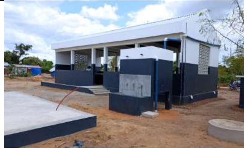
Picture 10 shows isometric view of newly constructed market in Guara Guara Buzi
