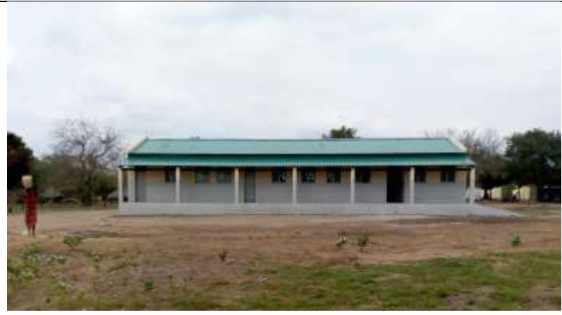
Picture 8 shows that the newly constructed school block-2 with gender friendly toilet backside the school in Chicuacha, lot1, Chibabava district.
