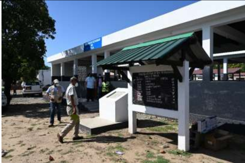
Picture 1 shows front view of newly constructed markets in Tica, Nhamatanda
