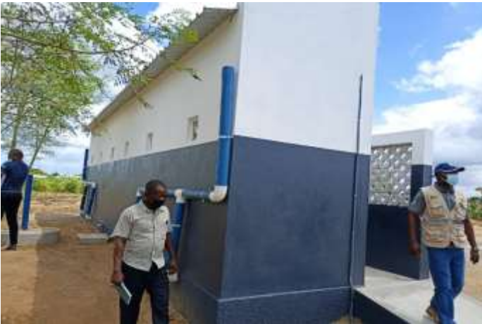
Picture 11 shows newly constructed gender friendly toilet (back view) in Guara Guara Buzi
