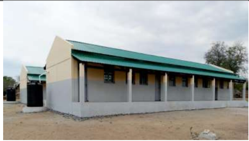
Picture 11 shows that the newly constructed school block-2 in Madombatomba, lot1, Chibabava district.
