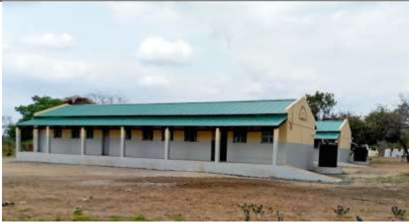
Picture 10 shows that the newly constructed school block-1 with gender friendly toilet behind the school in Madombatomba, lot1, Chibabava district.
